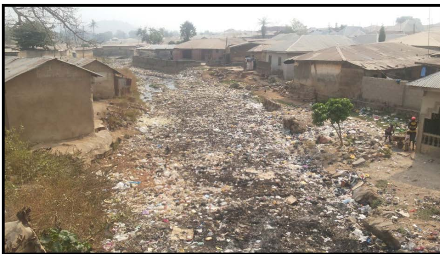
Image 1: Water channel filled with solid waste in Suleja Source: Authors' field survey
