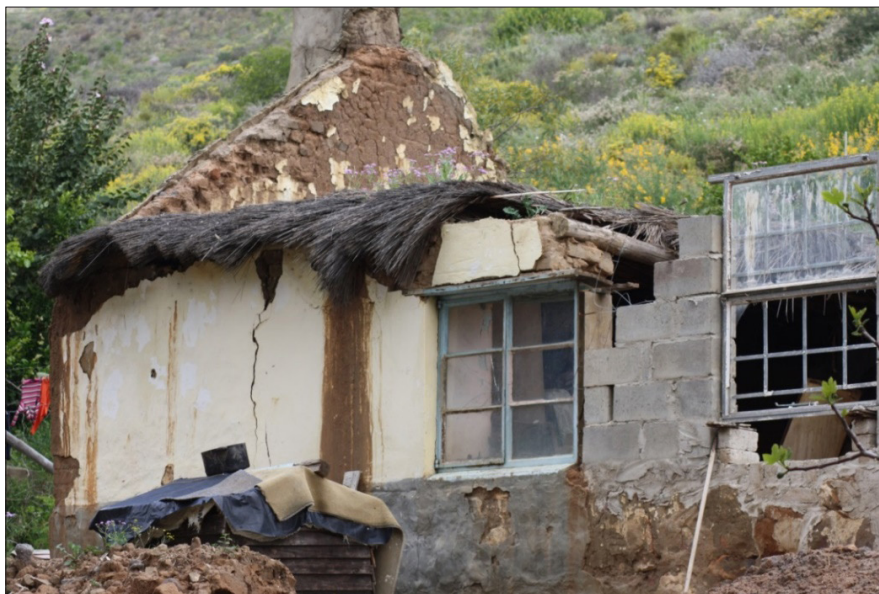
Figure 2: A dilapidated thatch cottage along the main road in the Kerk Straat precinct Source: Image by author, 2016
