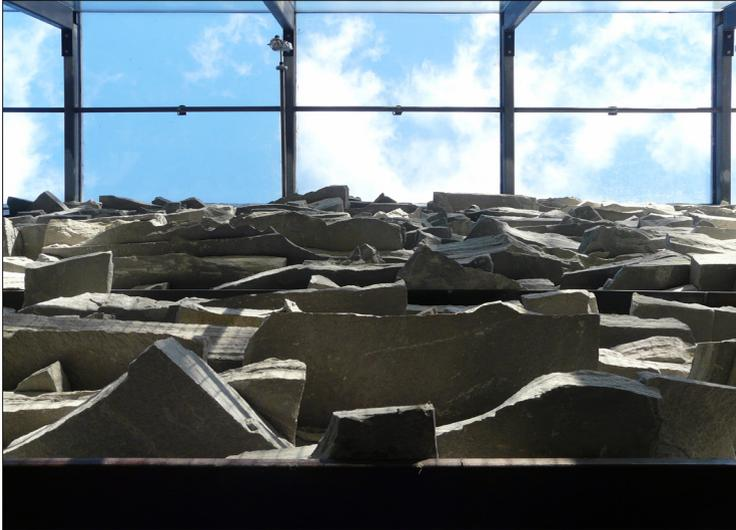
**Figure 12:** Elevated stacked stone wall acting as a light filter to the interior and the exterior glass wall providing thermal isolation (Auret).
