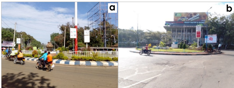
Figure 10a: Roundabout at Ang'awa Avenue and Jomo Kenyatta Avenue intersection (KIWASCO branding)
