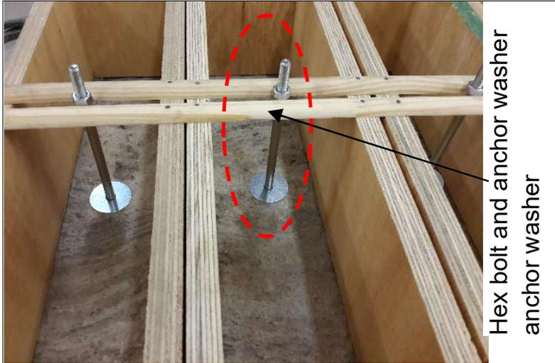
Figure 1: Timber box formwork
