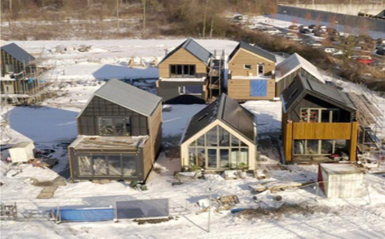
Figure 7: De Stripmaker, Almere, built using Wikihouse panels
