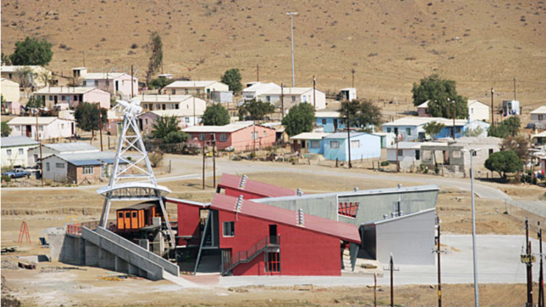
Figure 4: The David Klaaste Multipurpose Centre (now the THUSONG Centre) Source: CS Studio Architects, 2021
