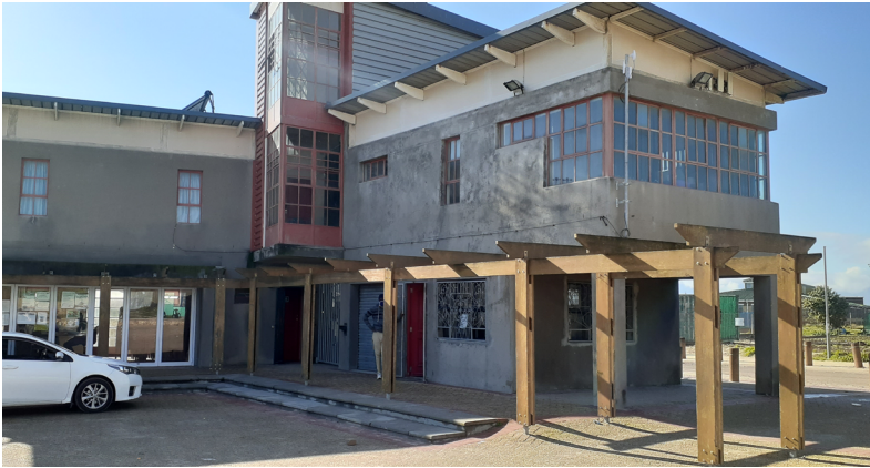
Figure 14: Active Box used as councillor's office Source: Image taken by author
