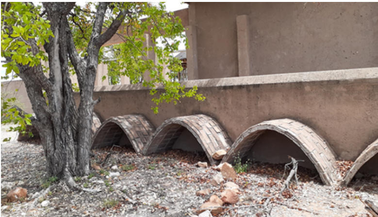
Figure 9: Vaults constructed by EPWP vault builders in training Source: Image by author
