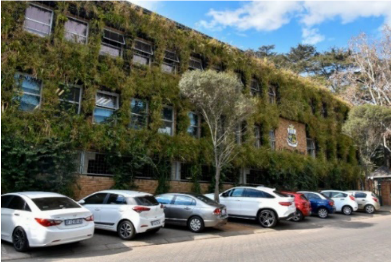
Figure 2: The veld wall of the Keyes Art Mile, Rosebank, has created a novel precedent where “wild” Egori grassland species were planted in a Gro-Wall system retrofitted to a brick façade. The wall alleviates the sun’s glare and heating produced on the northern and western façades and creates a unique ambience along the street that houses many art galleries. Source: Images taken by Author, 2018
