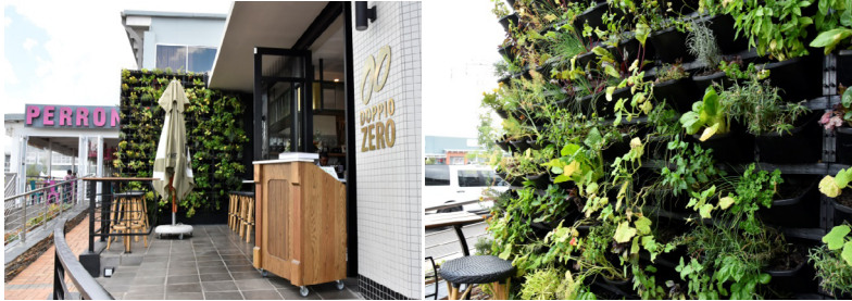
Figure 3: The edible green wall at Doppio Zero, making use of the Gro-Wall system for exterior conditions on a northern aspect Source: Images taken by the author, 2019
