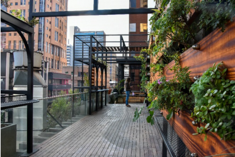
Figure 5: The greening strategy of the Neighbourgoods Market, with galvanised steel gutters fixed to steel frames and clad with timber slats, bolted to the frames. The wall provides fresh herbs for use at the market and for customers to experience and enjoy in their ciders Source: Images taken by the author, 2020
