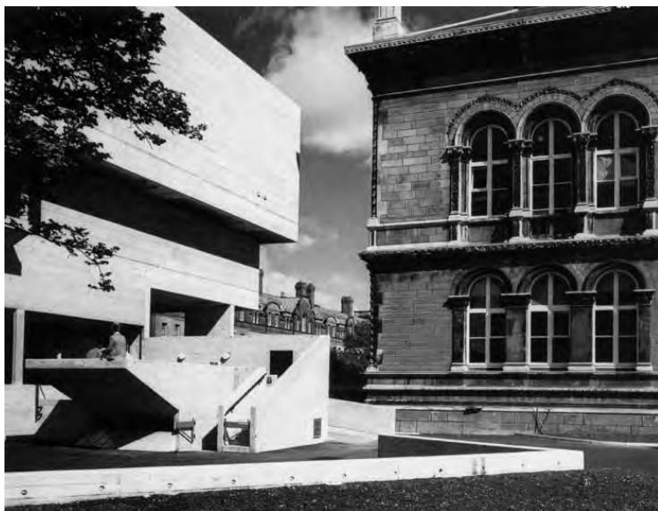
Figure 3: Trinity College Library, Dublin. The modernist block is an extension of the collegiate tradition of a quadrangular disposition of buildings.
