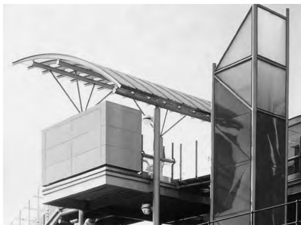
Figure 7: Dockland Light Rail Station. Designed to be used as a kit of parts for all stations.
