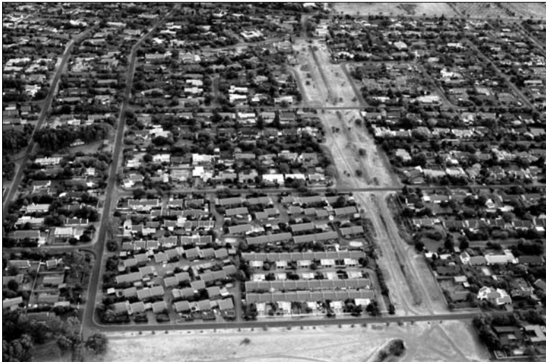
Figure 4: Open spaces as a trench for storm water Source: Steyn & Schoeman 2006: CD- ROM
