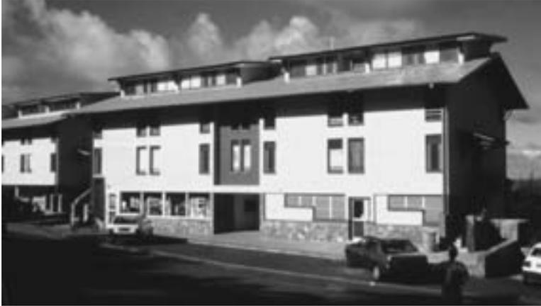
Photo 2: Contemporary three storey block of flats of Compressed Earth Blocks on the Island of Mayotte
