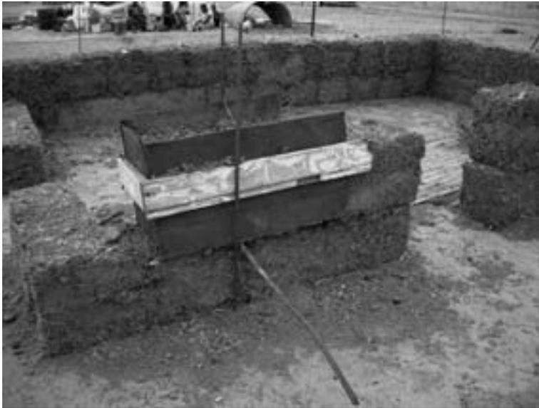
Photo 4: A mix of cob and straw-clay technique near Harrismith in the Free State
