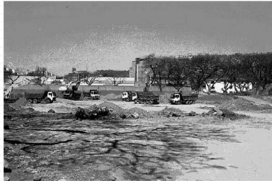
Photo 1 : Inner-city infill development adjacent to Sunnyside: the DTI campus development
