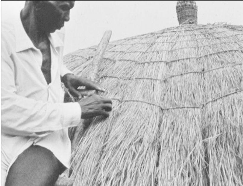
Figure 4: Construction of the first grass dome house under the supervision of Mof Mota, aged 85, in 1979. Photograph by the author
