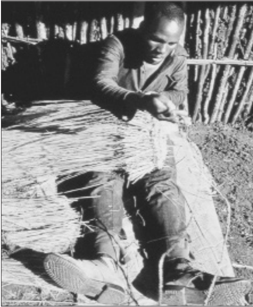
Figure 5: John Thubana Mnguni weaving the ' isiqongolo ', the crown of the grass dome house. Photograph by the author.
