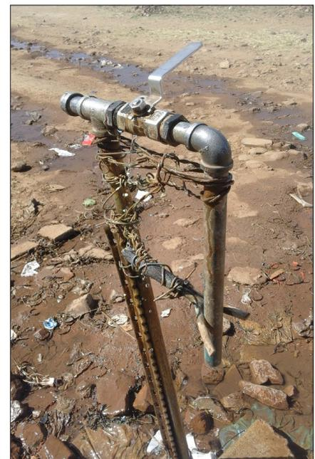
Figure 4: A leaking tap fixed with a forked stick and barbed wire
